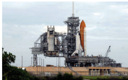
Launch Pad 39-A Cape Canaveral, Florida (1965)
